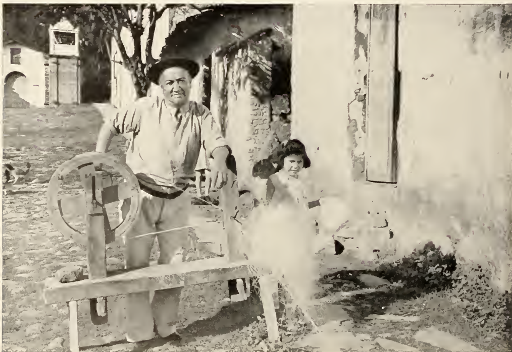
FIGURE 12.—Small machine for spinning letona fiber into yarns or twines. El Salvador.
