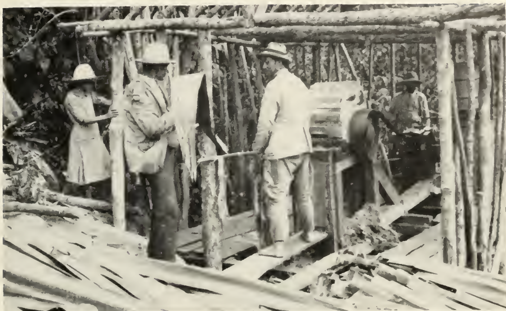
FIGURE 32.—A mechanical defibrator, or raspador, made in Colombia. It has a capacity of about 110 pounds (50 kilos) of fique fiber an hour. Photograph from Sr. Adel López Gómez, of the Ministry of National Economy of Colombia.
