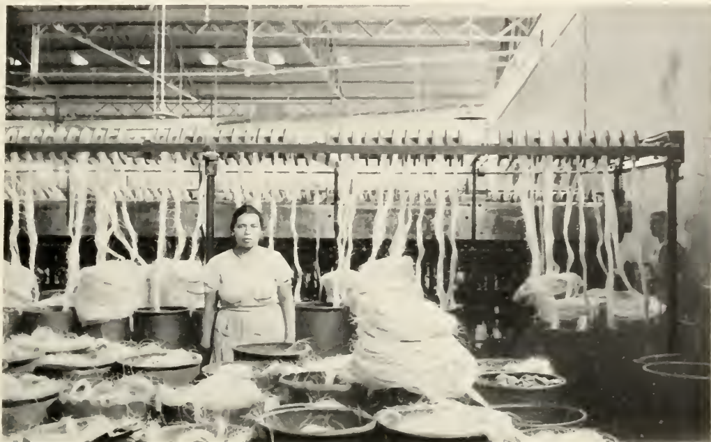
FIGURE 13.—Interior of a factory for preparing letona fiber ("Salvador henequen") for spinning into twines. El Salvador.
