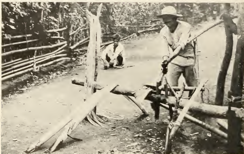
FIGURE 46.—Stripping abacá by pulling the tuxie under a serrated knife pressed against a block of wood by means of a spring pole. Province of Albay, P. I. Photograph from Philippine Bureau of Science.
